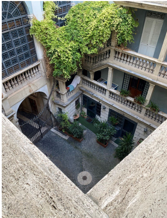
Figure 1 The office courtyard
