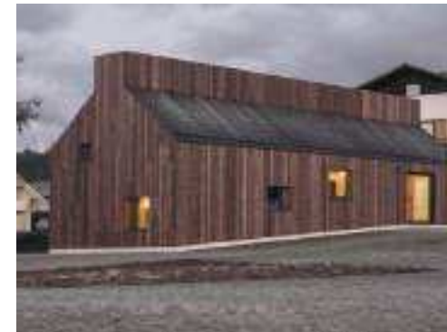
Dekleva Gregoric-Chimney House
