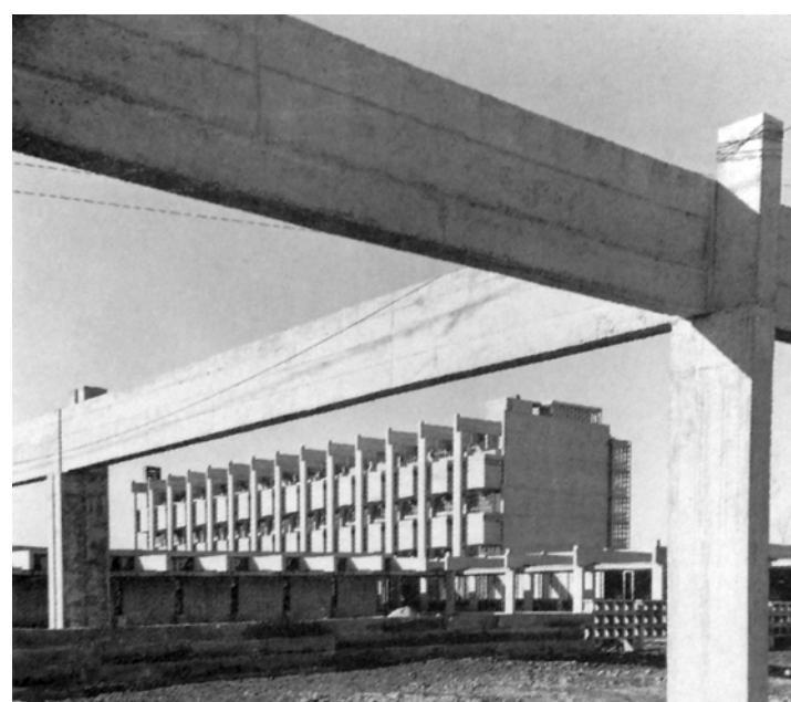
Exterior space defined by structure
